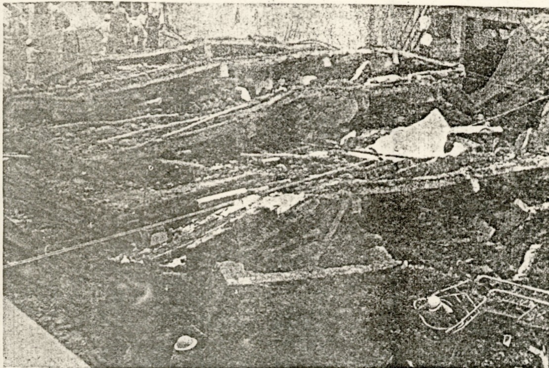
A sandwich of concrete: The seven floors came down like a pack of cards killing about 100 people
